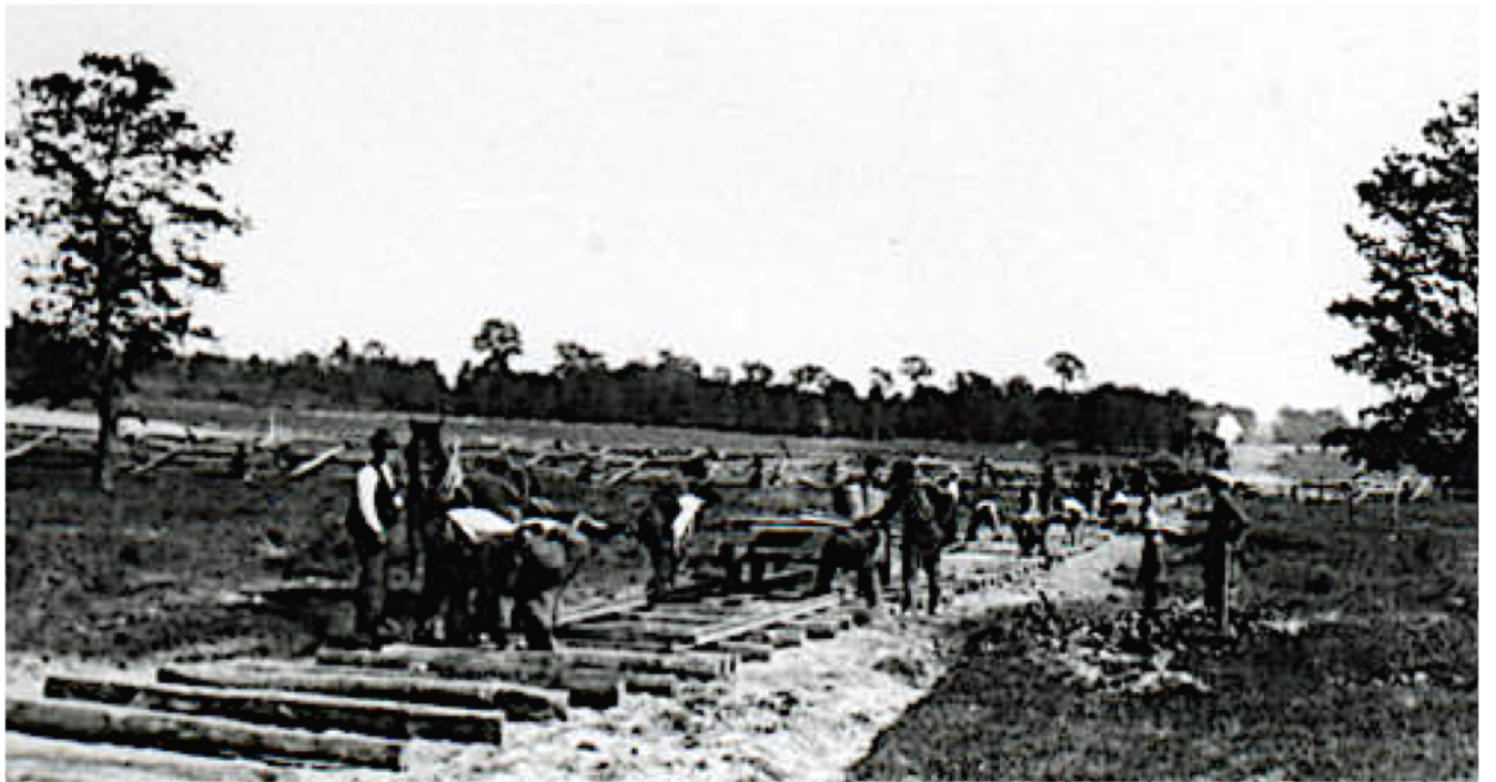
Construction of Interurban Line to Gates Mills
